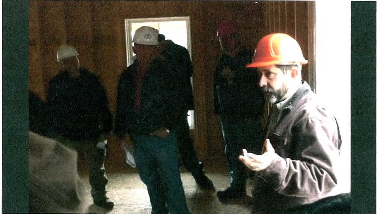
Stephen Berko explains the intricacies of a building under construction to NCC students Monday.
